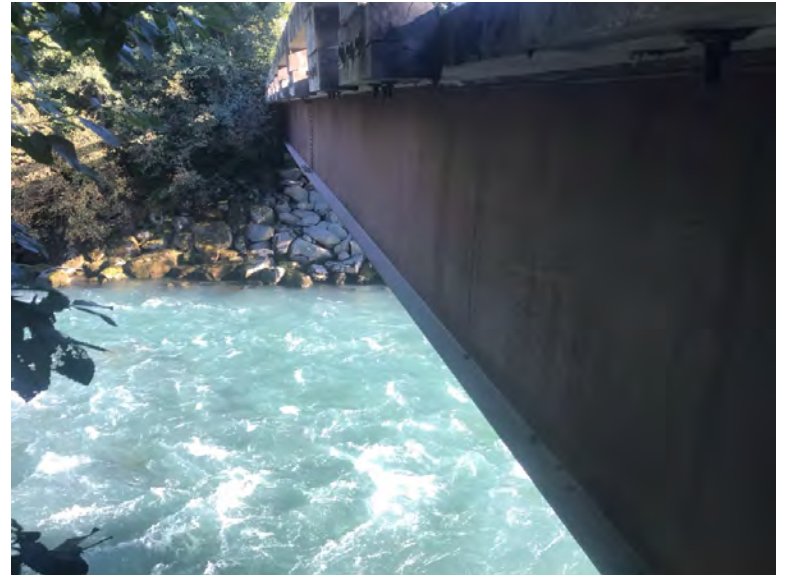
Left Bank Abutment when facing downstream
