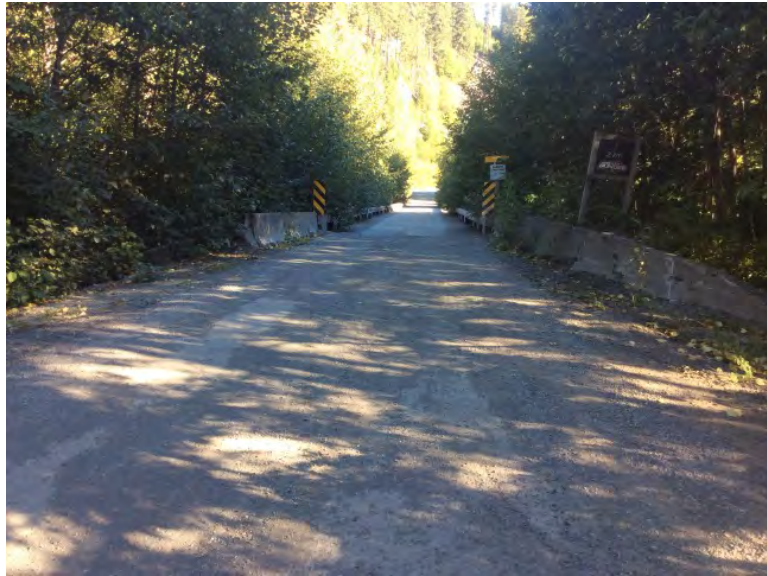
Approach from Right Bank when facing downstream
